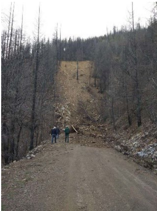
Figure 2 Fillslope failure from a road higher in the watershed onto a road in the Walker Creek watershed in Klamath National Forest, winter of 2015 after the 2014 Happy Camp Complex Fire
